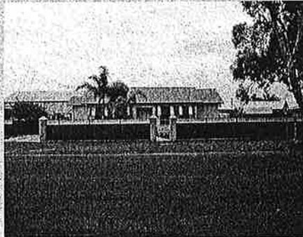
View of No. 25 Barwan Street
