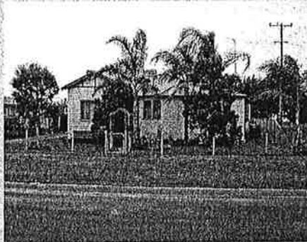
View of No. 29 Barwan Street
